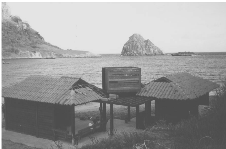
Figure 3— Example of a “PIC”, where is observed the modulation and its insertion in the natural environment. It is important to see some constructive elements such as pillars, coverings and wooden bench - they will be repeated in other built elements.
